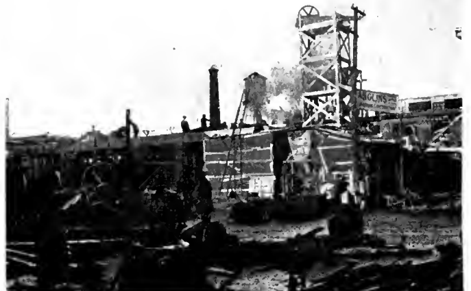
Concrete for first floor being poured—Feb. 19, 1916.
